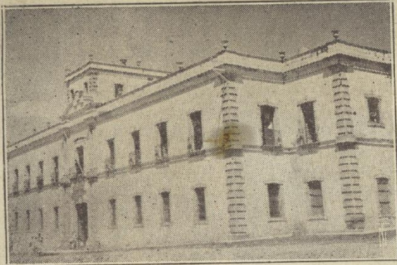
Fachada del Hospital General "SAN FELIPE"
